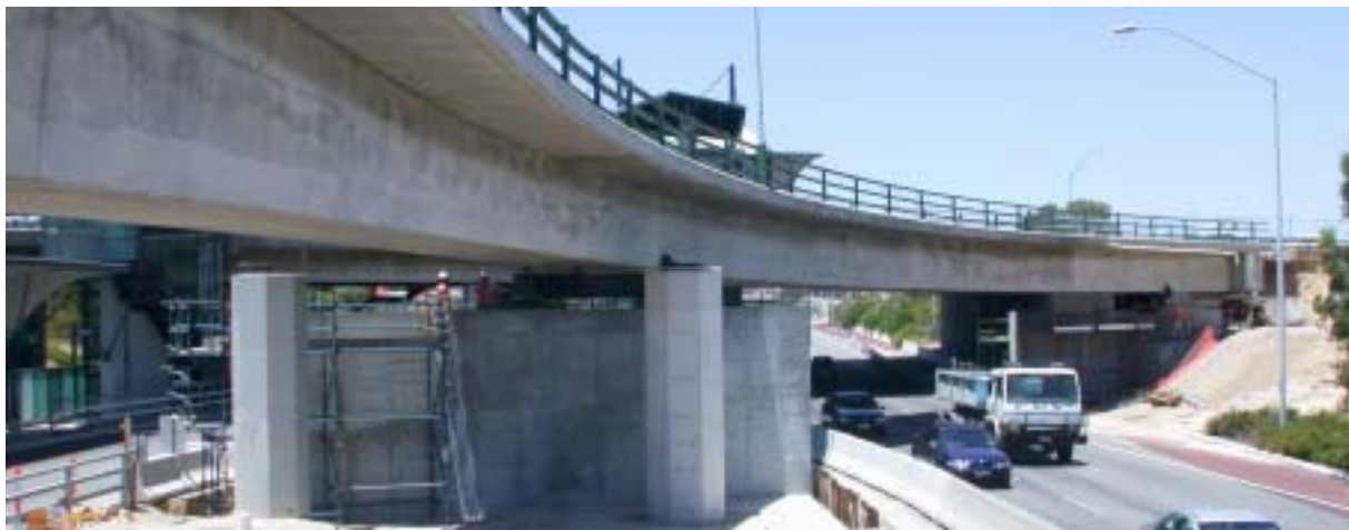
Figure 8: Bridge #1295 Nearly There!!!
