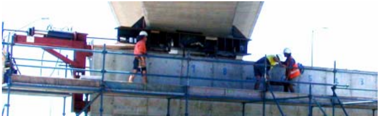
Figure 7: Support Cradle and Horizontal Jacking System at TS2
